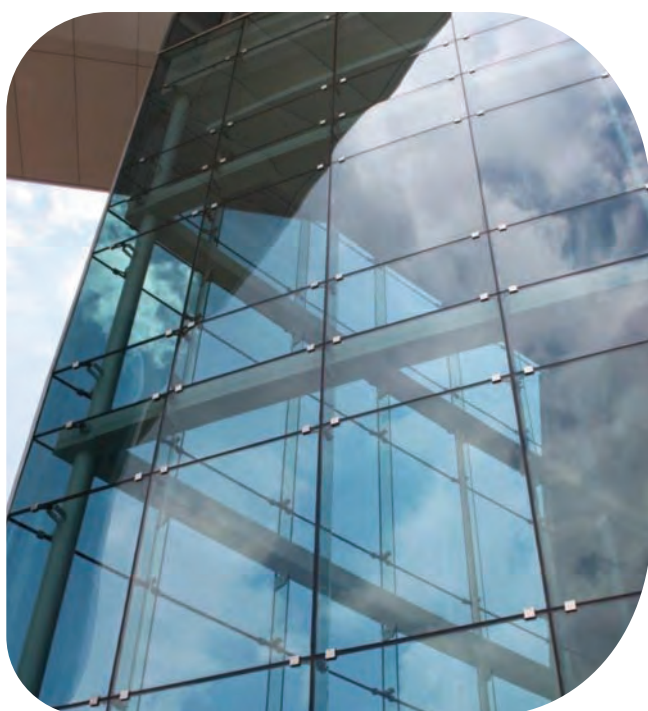
Pilkington Solar – E Bluegreen Telesure Headquarters, South Africa Photo compliments of Pilkington
