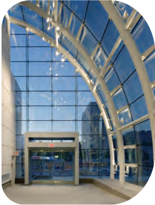
West Midtown Ferry Terminal, New York.
